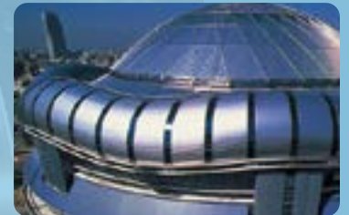
Roof of a dome
