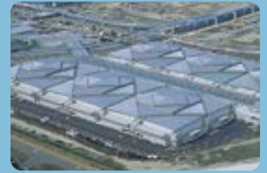
Roof of a building
